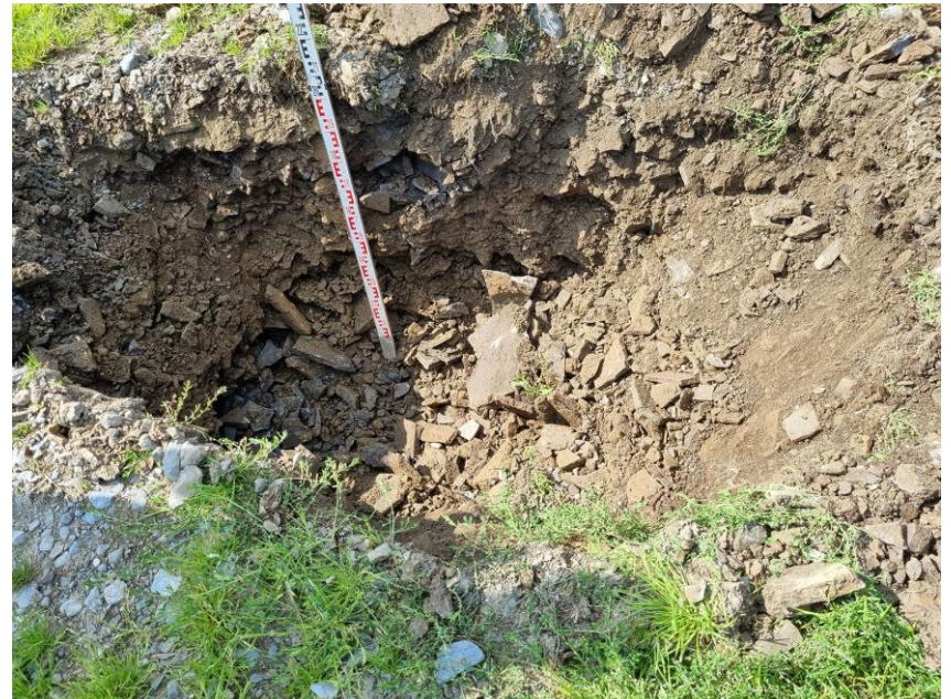
Trial Pit at Ballyring
